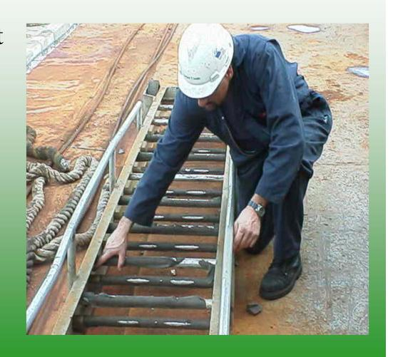
Inspect before use for cracks, dents, and missing rungs.
