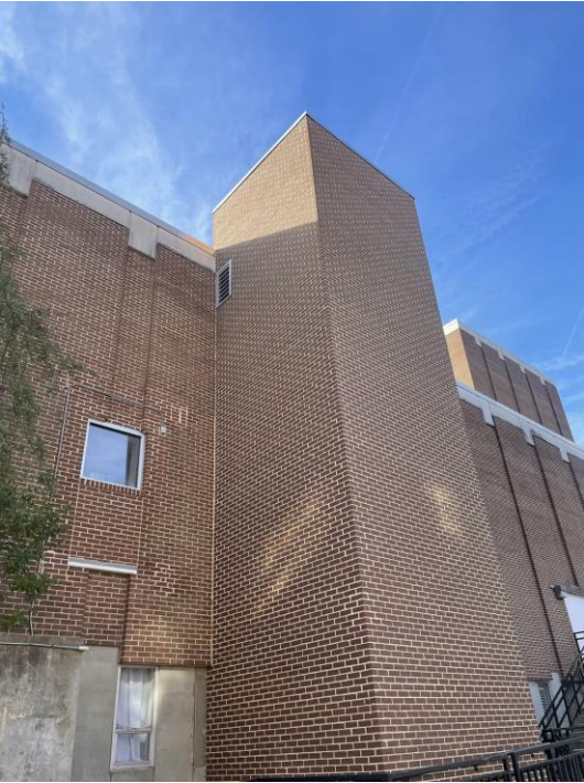
Existing elevator addition
